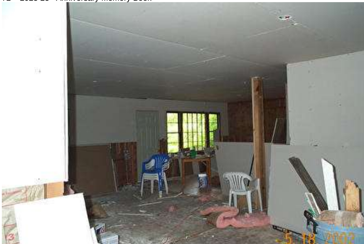
Figure 108 – 2002 – Construction – Drywall And Work Table
