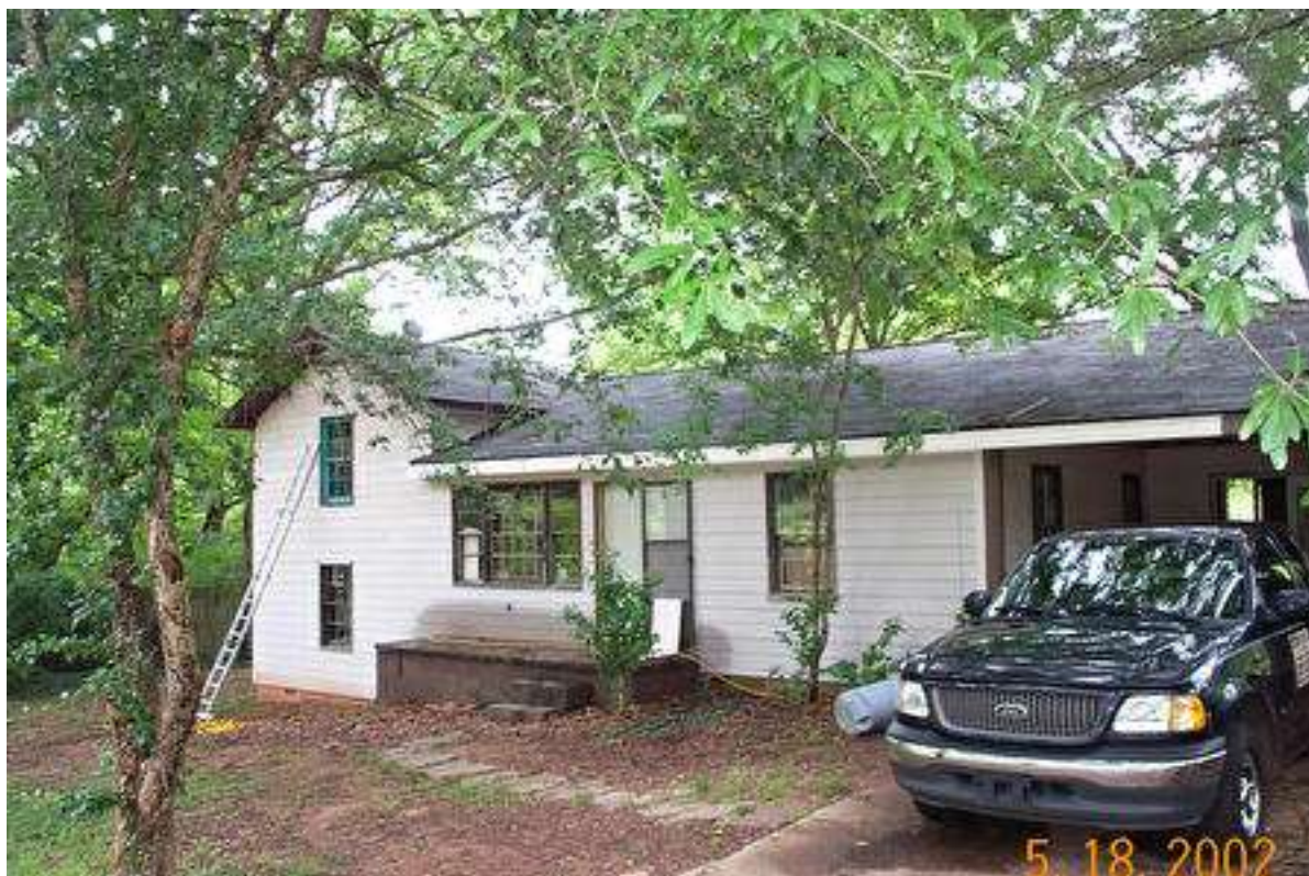
Figure 109 – 2002 – Construction – Front Of the House
