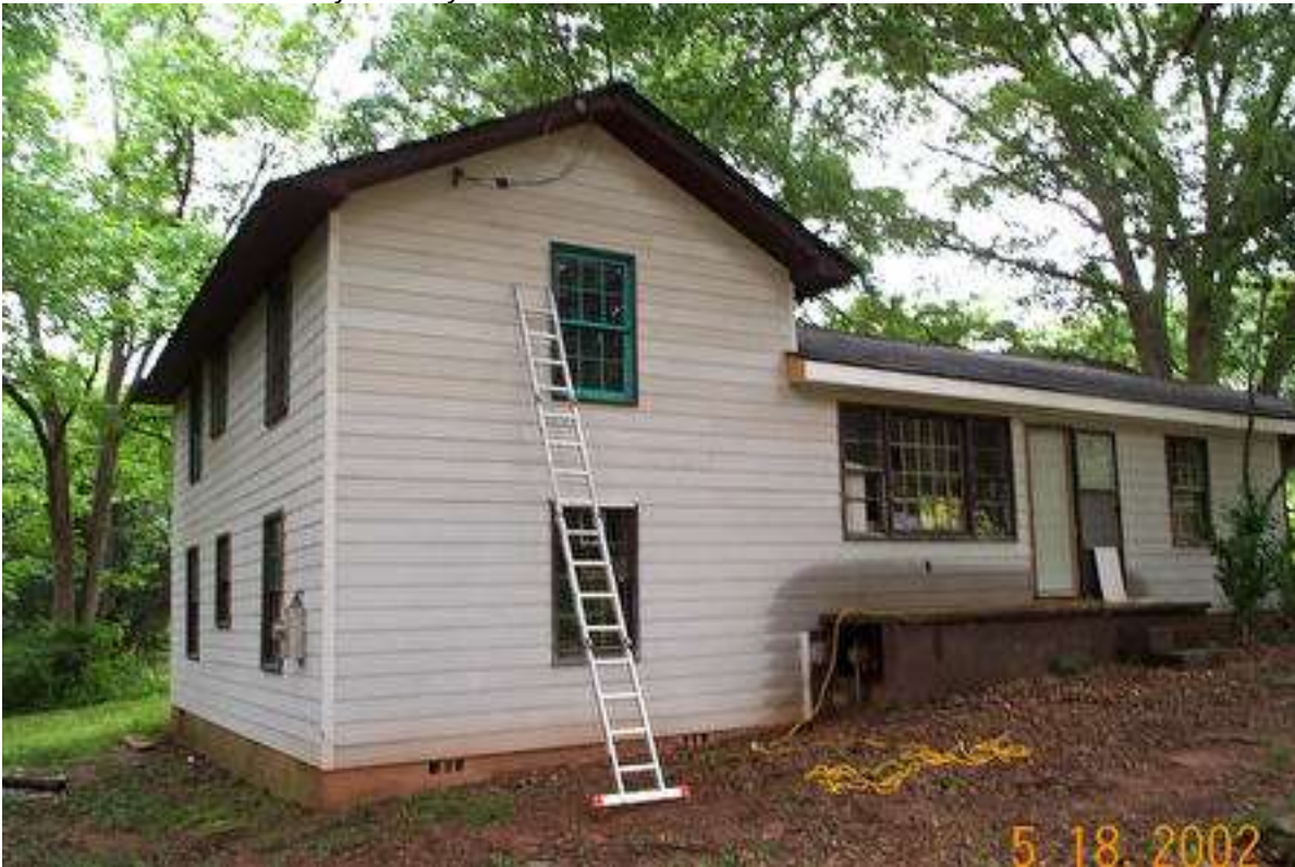
Figure 110 – 2002 – Construction – New Siding
