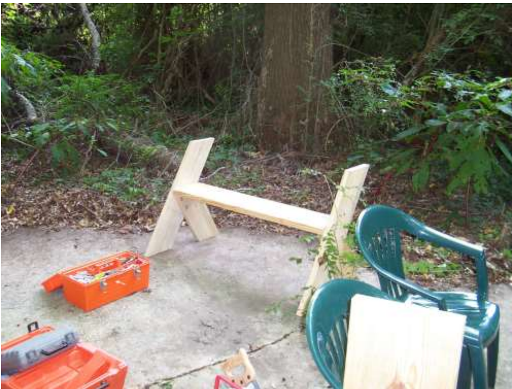
Figure 207 – 2004 – Leopold Bench – Nearly Finished Bench
