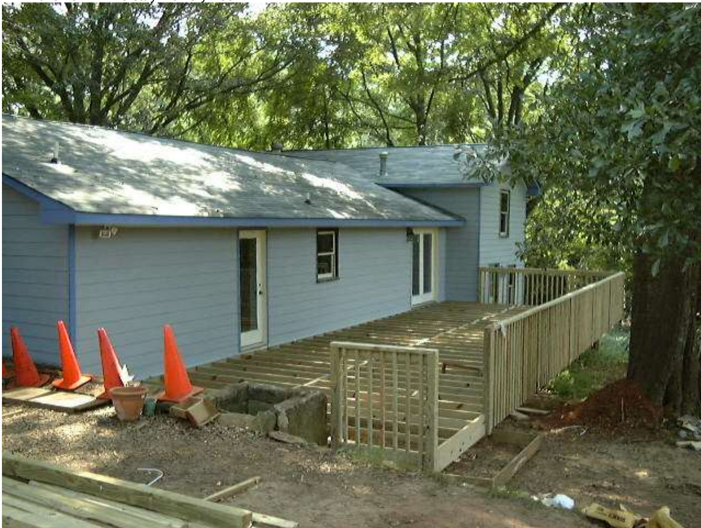
Figure 112 – 2002 – Construction – New Deck
