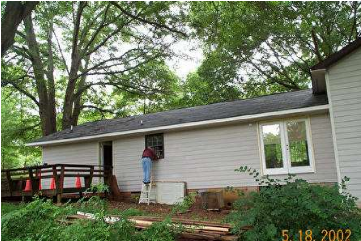
Figure 111 – 2002 – Construction – Back Of The House (Old Deck)
