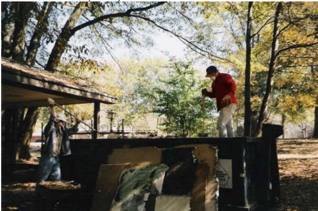
Figure 60 – 2000 – Construction – Full Dumpster
