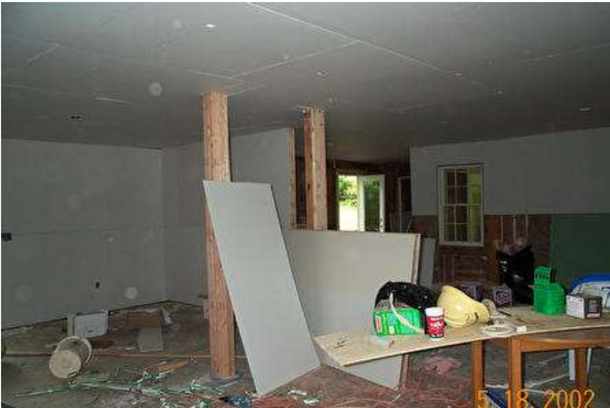
Figure 107 – 2002 – Construction – Drywall And Work Table
